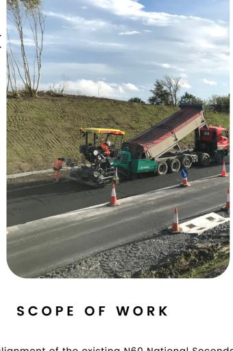
Realignment of the existing N60 National Secondary Route comprising the construction of a Type 2 single carriageway road for a distance of approximately 1.4 km.
